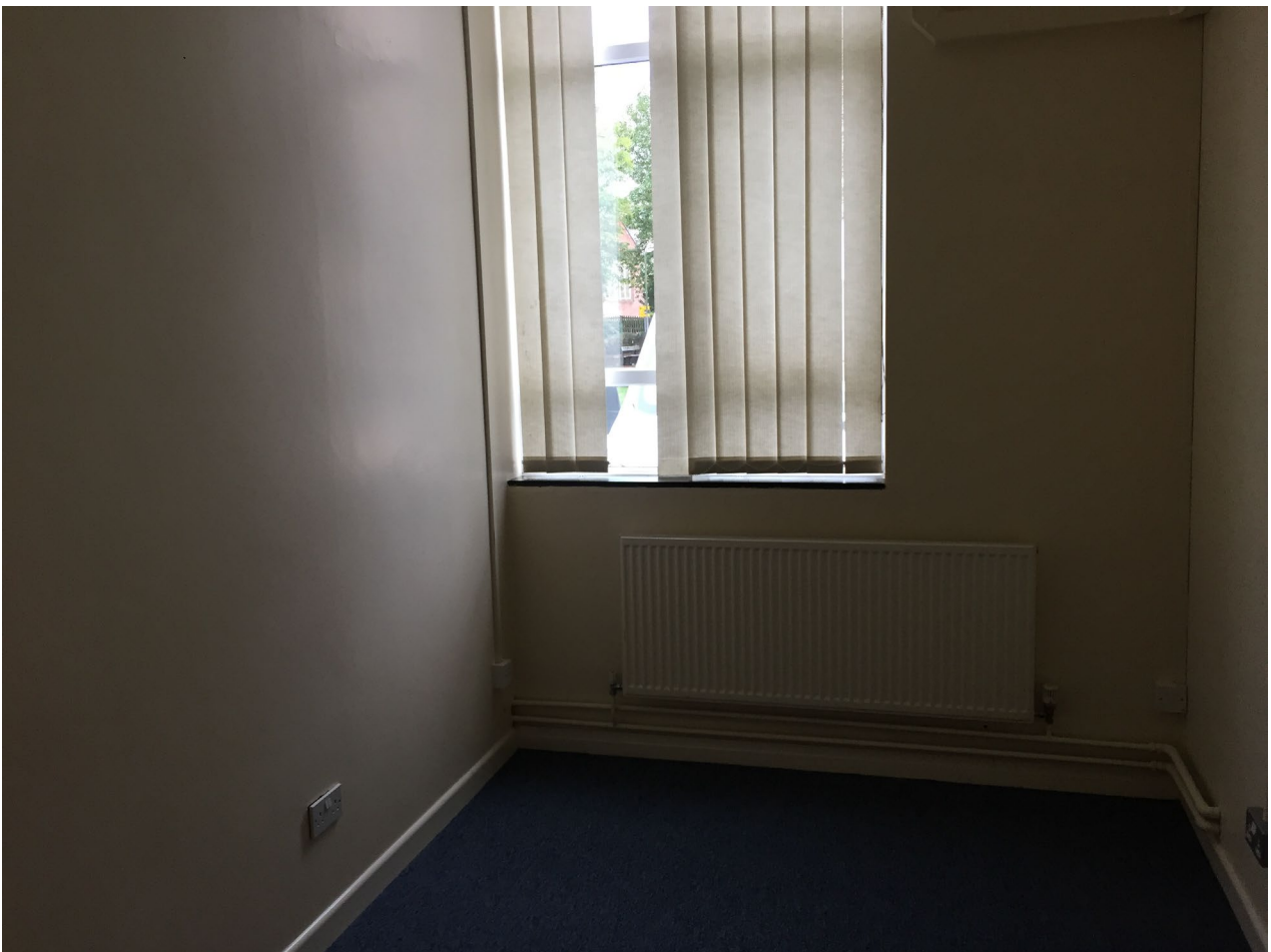
View from within the property
