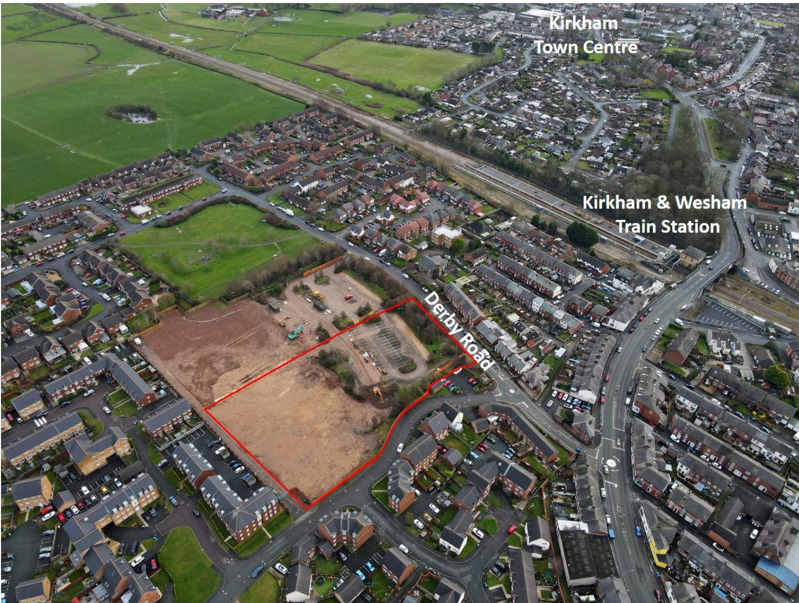
Photo of the Property looking south east (red line for identification purposes only)
