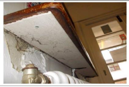
Cement removed and replaced with modern insulating board Notes
