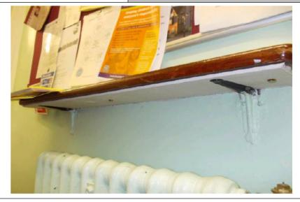
Notes Cement panel removed and replaced with modern insulating board
