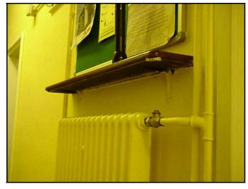
4.2 Asbestos cloth insulation
