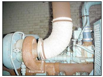
**4.3** Asbestos gasket to pipe flange
