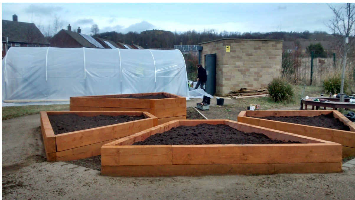
Figure 5 Construction of the Houghton-le-Spring Community Garden
